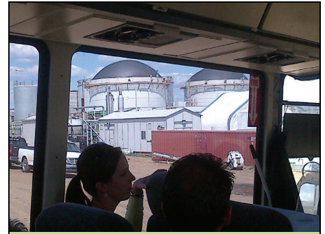
The manure bio-digestors in operation, showing their peaked dome.
